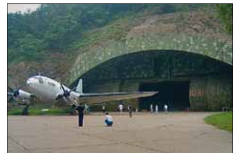
The underground hangar complex at Luyang / Rhange-Zhen is no longer in operational use, and was never completed. It is unusual as it includes tunnels sized for Badger and Beagle bombers. The segmented blast doors were built to resist near miss nuclear attacks. The very recent upgrade of the Hainan Do airbase yielded a similar configuration.
