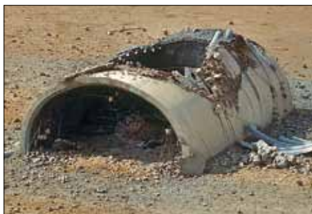
The survivability of Iraqi HAS varied widely. The least robust HAS were destroyed with single rounds, others required multiple hits. Depicted HAS at Al Salem.
