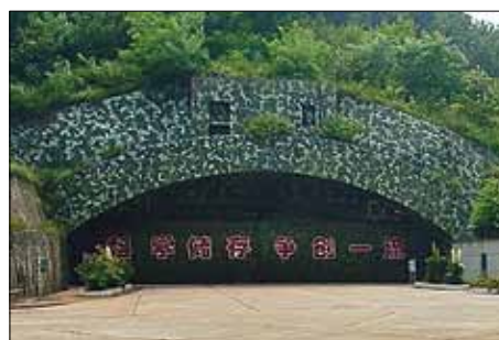
The underground hangar complex at Luyang / Rhange-Zhen is no longer in operational use, and was never completed. It is unusual as it includes tunnels sized for Badger and Beagle bombers. The segmented blast doors were built to resist near miss nuclear attacks. The very recent upgrade of the Hainan Do airbase yielded a similar configuration.
