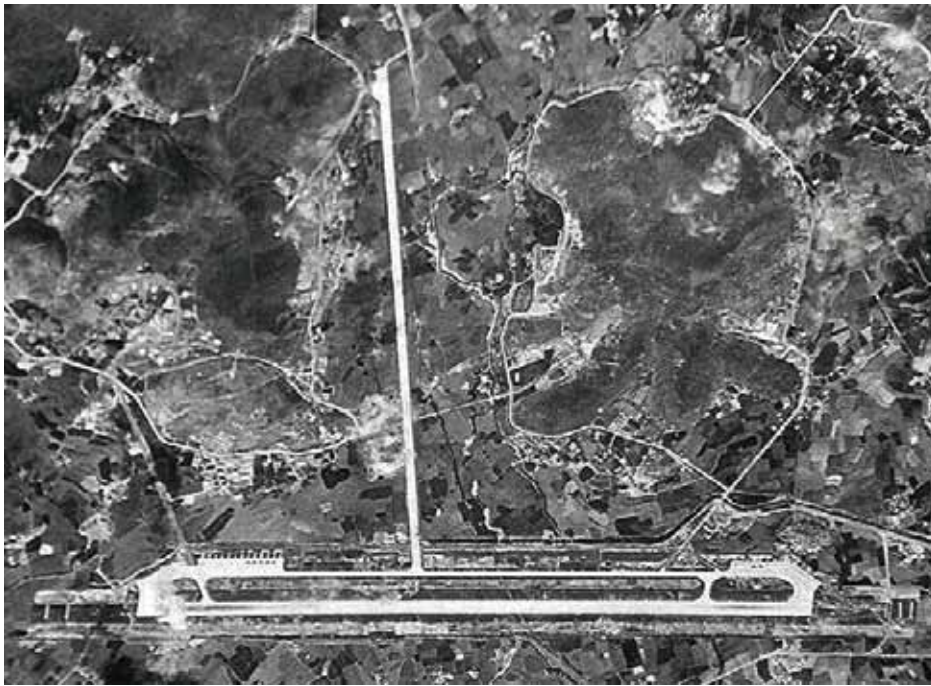
1962 KH-2 Corona satellite image of the PLA An Ching airbase under construction. The wide taxiway north of the runway complex is used as an auxiliary takeoff only runway for aircraft, and connects to the apron in front of the primary tunnel entrance. Yet to be constructed is a taxiway to the east of the complex, to a second tunnel entrance.
