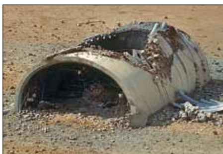
The survivability of Iraqi HAS varied widely. The least robust HAS were destroyed with single rounds, others required multiple hits. Depicted HAS at Al Salem.
