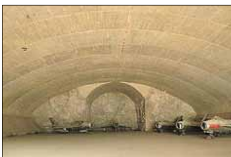
The underground hangar complex at Luyang / Rhange-Zhen is no longer in operational use, and was never completed. It is unusual as it includes tunnels sized for Badger and Beagle bombers. The segmented blast doors were built to resist near miss nuclear attacks. The very recent upgrade of the Hainan Do airbase yielded a similar configuration.
