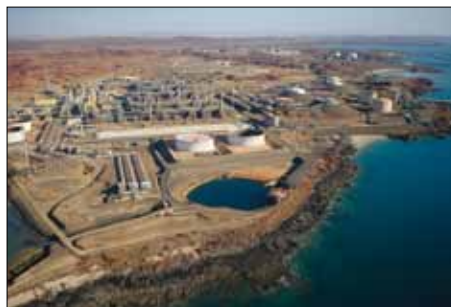
Woodside Burrup Peninsula plant.
