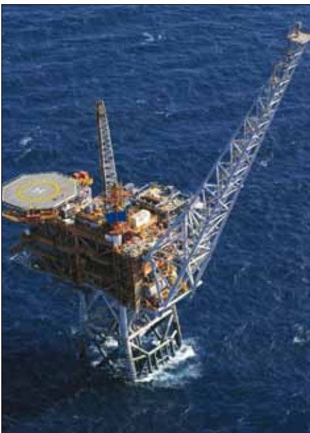
Woodside Pluto production platform.
