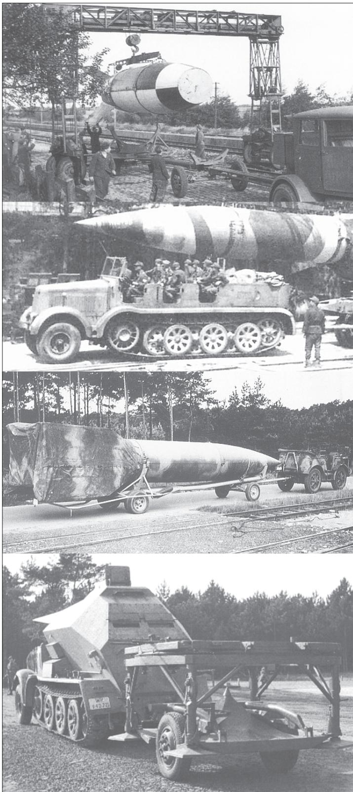
Battery support equipment for the A-4, top to bottom: Strabo mobile gantry crane for transloading, Sd.Kfz.8 12 tonne halftrack tow tractor, Vidalwagen transloader trailer, Feuerleitpanzer launch control centre towing the launching pad.
