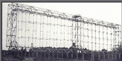
Knickebein transmitter ground station. Many were built along the coast of occupied Europe.
