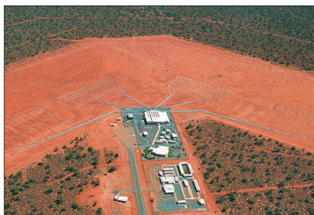
JORN project transmitter site, Laverton WA. (Photo: CPL Dave Broos, Defence Public Affairs)
