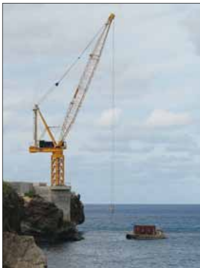
Norris Point container facility at Christmas Island (© Commonwealth of Australia 2011).
